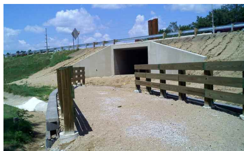
Approach to U.S.20 tunnel, looking north, Aug. 6, 2010
